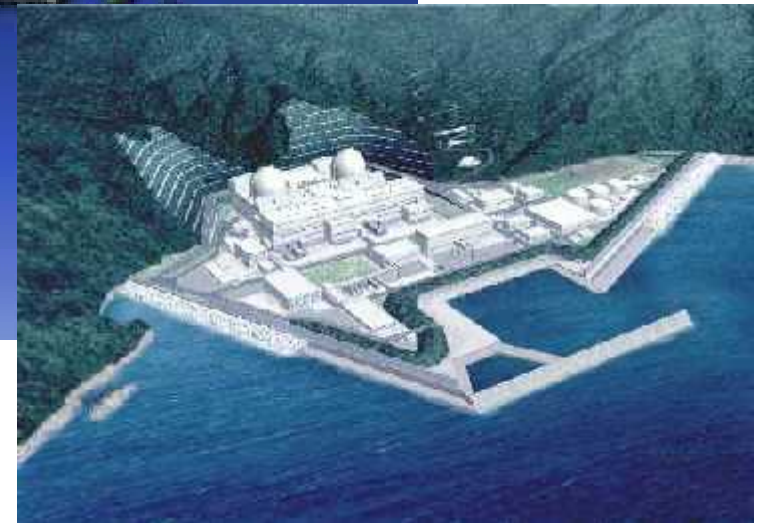
Tsuruga Plant No. 3, 4 (preparing for construction)
